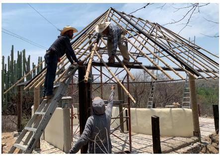
Miguel and Catalino designed a new structure combining metal and ocotate (a large diameter bamboo) and also added four new pilars of metal and concrete. This structure should easily last 50 years. Putting up the new structure took a good two months. Since then the team plus a few parttime workers have been putting on the palm. The palm should last 18 to 20 years.
